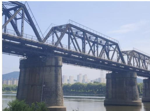
Figure 2: Actual picture of the bridge
