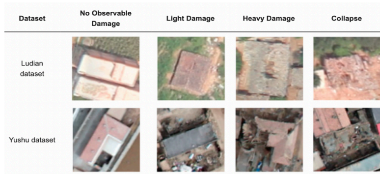
Figure 2. Sample of damaged buildings from each class in both earthquakes (Lin et al, 2019)
